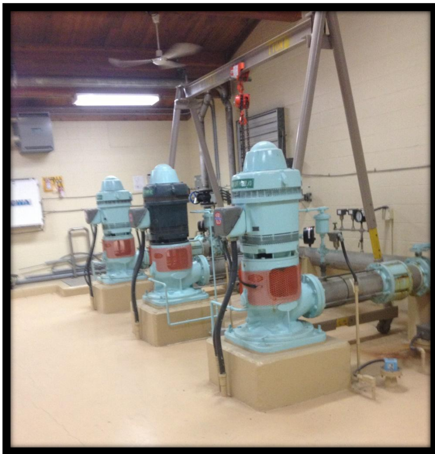
Figure 6 :Elk Lake Water Treatment Plant
